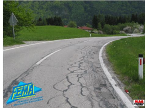
Longitudinal road ridges caused by heavy goods vehicles, road settlement or road repair can be very hazardous to motorcyclists. Hazards often occur in connection with resurfacing work. Longitudinal road ridges of more than 2cm should always be tapered. If not possible to remedy immediately, motorcyclists should be warned of hazard by appropriate traffic sign and longitudinal road ridges should be marked with cones.
