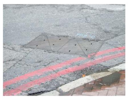
after a short period of time (possibly as little as a month of normal wear), these covers can give a grip of around 0.5, which is still more than adequate for use on a flat, straight piece of road with no junctions. After 12 months, however, the grip has deteriorated to 0.3, far below the minimum expected from the surrounding road surface. The covers are not designed to maintain grip.
