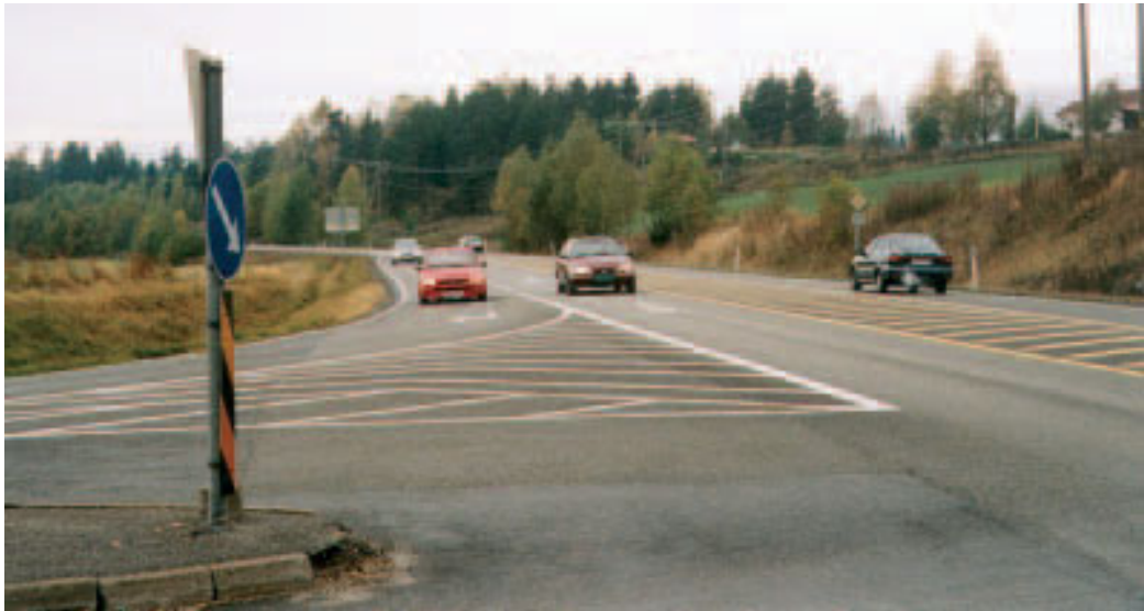
Rv 35 Vikersund. A large vehicle in the turning lane can hide a motorcyclist in the through lane.
