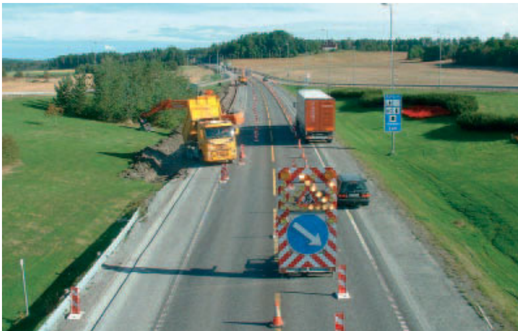
Picture of sections where roadwork is ongoing
