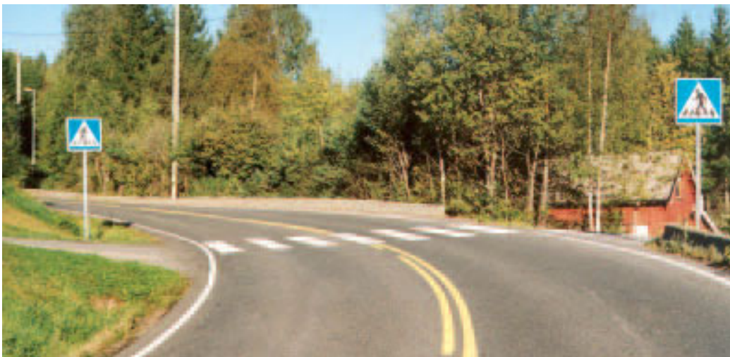
Pedestrian crossing on a curve is a poor solution both because motorcyclists may skid on the slippery markings and because the visibility relative to crossing pedestrians and cyclists is poor.
