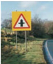
The use of a yellow backing board undoubtedly increases the visibility of this sign but also adds to the visual intrusion. Such signs should be used very sparingly, both to retain their impact and to
