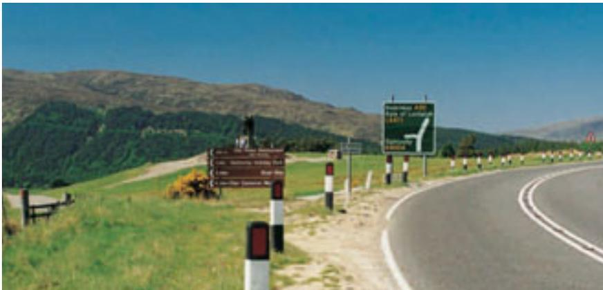
These signs have developed in an *ad hoc* fashion. The tourist sign is not easy to see and partly obscures the view of the Commando Memorial. The large advanced direction sign breaks the skyline and the sign forbidding parking on the verge may well be redundant. The verge marker posts are also visually intrusive and the roadside edge is worn and unattractive. The following sketches suggest alterations with different implications.
