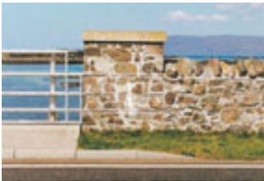
A well executed junction where the stone pillar connects the wall and fence simply and unobtrusively.
