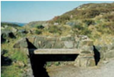
A good example of a seat at a lay-by constructed from squared timber and local stone, incorporated into the hillside.
