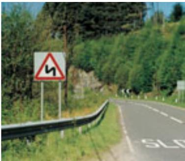
This sign has two poles and a backing board that help to increase its impact in this small-scale landscape. The two fixings help to prevent the sign turning in strong winds. A simple triangle sign could, however, be mounted on a single square section pole instead.
