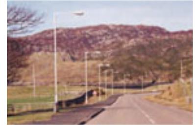
These lighting columns, along a stretch of road leading into a village, spoil the view of the hills beyond. If lighting is needed, perhaps fewer and lower columns should have been used instead.
