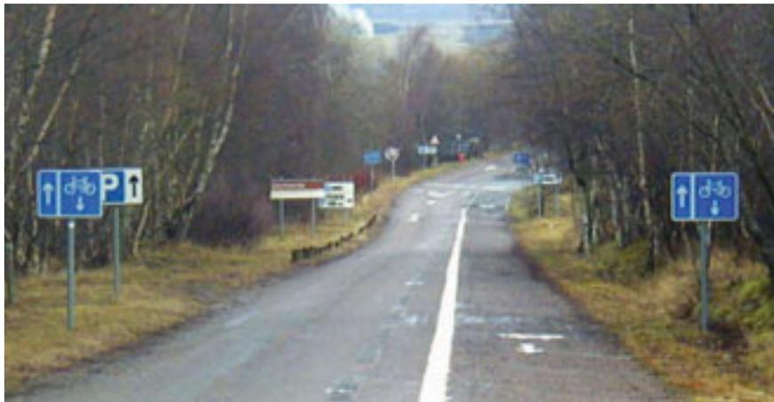
In this example a lot of new signs, provided where a contraflow cycle route is associated with a one-way road, have created a very confusing and intrusive effect.
