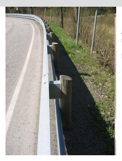
New guardrail design protects sub-rail against impact of snow plough
