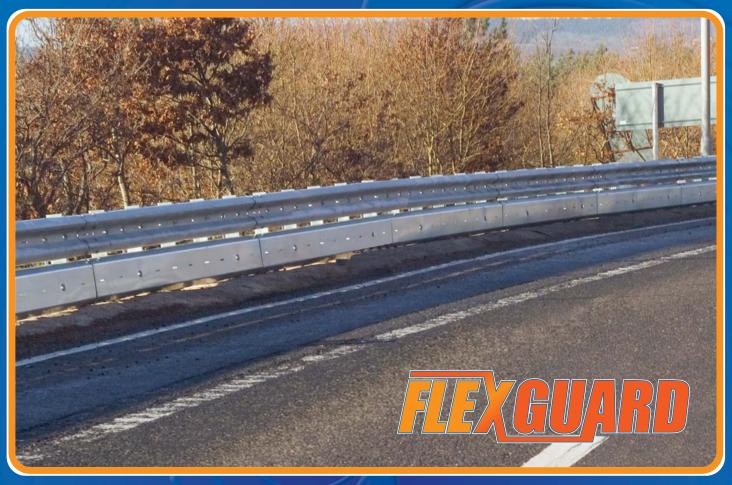
FLEXGUARD is a single sided retro fitted barrier system designed to protect motorcycles from travelling beneath road side barriers.
