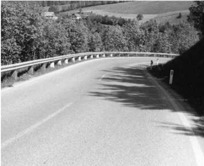
An Austrian road with a crash barrier fitted with CBP polystyrene impact attenuator
